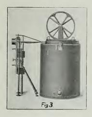
The large tank in the cut is filled with transformer oil and not only provides for a cooling effect on the bulb and other portions of the apparatus but also acts as a high tension insulator. About 90° F. is the best temperature for operation, the lower limit being about 50° F.
